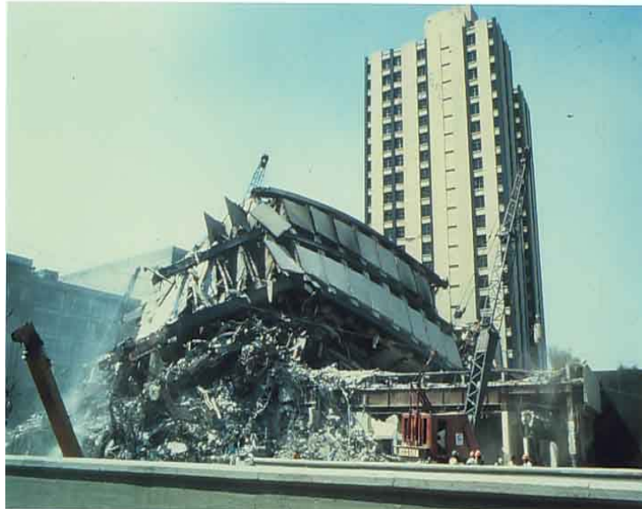
Front – 8 – Storied Building Collapsed Back – 15 Storied Building DID NOT (Mexico 1985)
