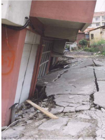
Fig.1 (a) Bearing Capacity Failures of Shallow Foundations in Adapazari (Yilmaz et. al. 2004).
