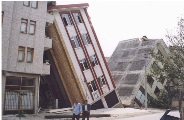
Fig 1(b) Bearing Capacity Failures of Shallow Foundations in Adapazari (Yilmaz et. al. 2004).
